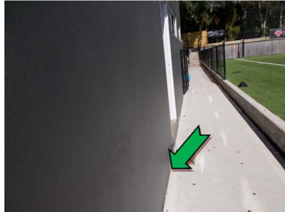
Photo 2. Exterior, ground level, ground, expansion joint – non asbestos-containing construction joint mastic.
