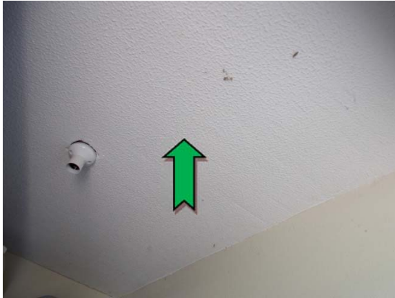
Photo 1. Exterior, ground level, ceiling – non asbestos-containing textured coating.
