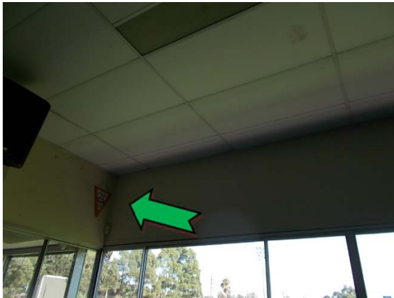
Photo 3. Interior, level one, north-west elevation, walls – non asbestos-containing compressed board.
