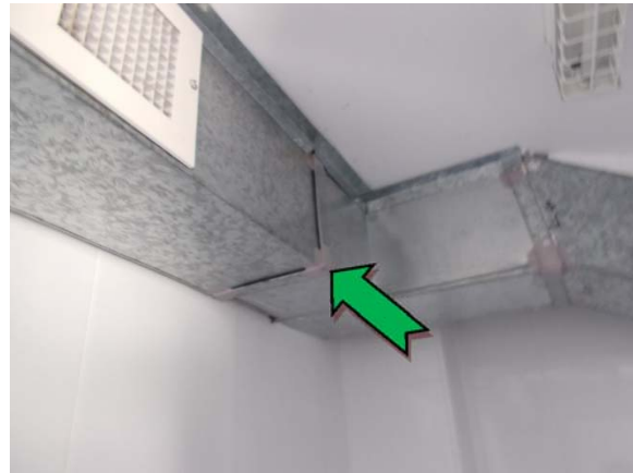
Photo 4. Interior, ground level, ceiling, duct work – non asbestos-containing mastic sealant.
